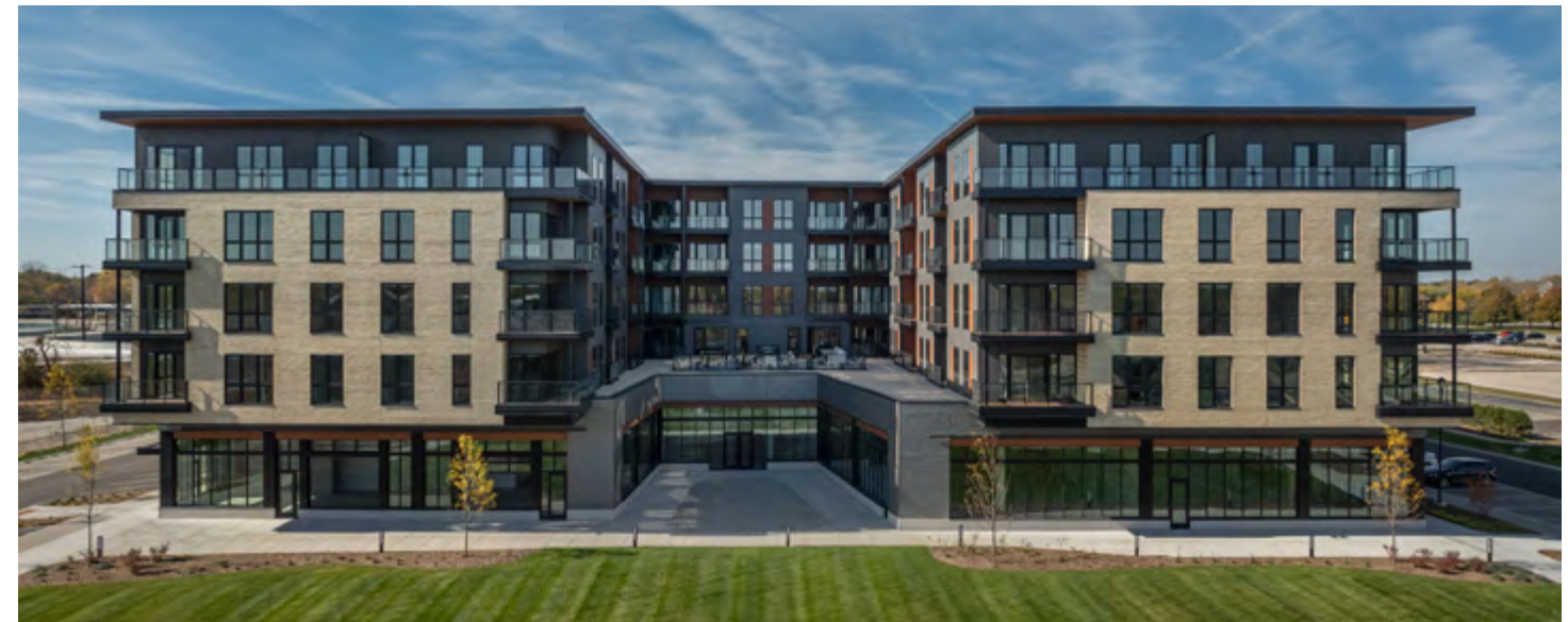
FIGURE 3.2.d: Example of successful exterior material integration
