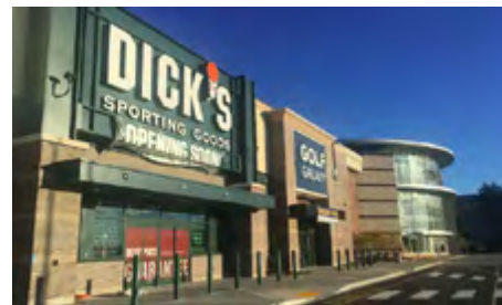
FIGURE 3.2.b: Recent Investment in the Mall Facade's
