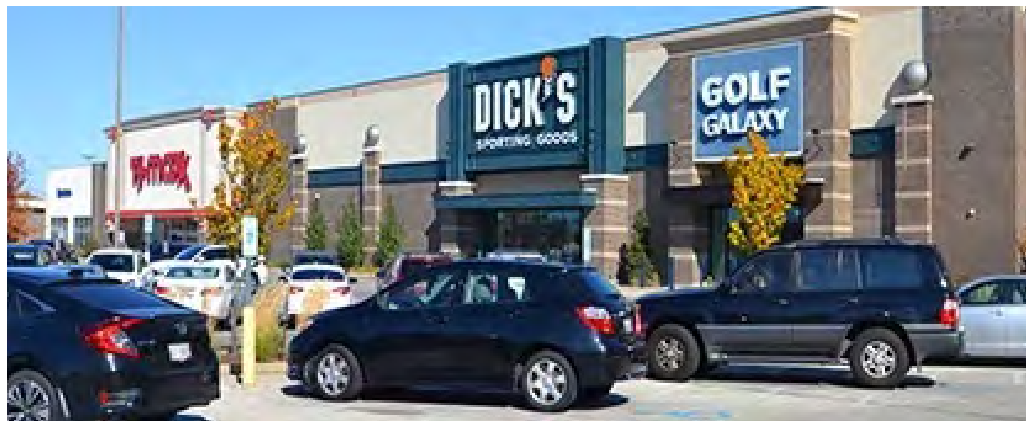
FIGURE 1.3.3.a: Recent Facade Renewal Along North Primary Tenant Space
