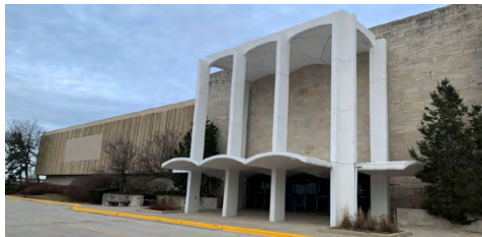
FIGURE 1.3.4.a: Vacant Boston Store Intended for Demolition
